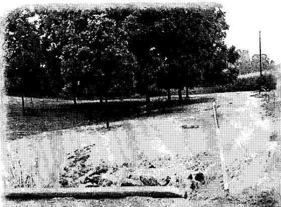
Stormwater runoff carrying sediment & other pollutants
