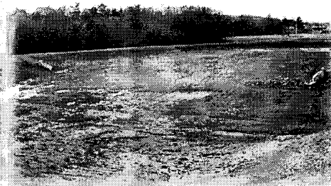
Stormwater detention basin
